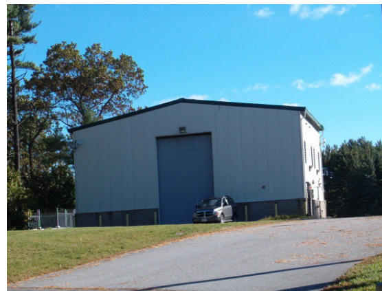
Cosgrove Disinfection Facility
